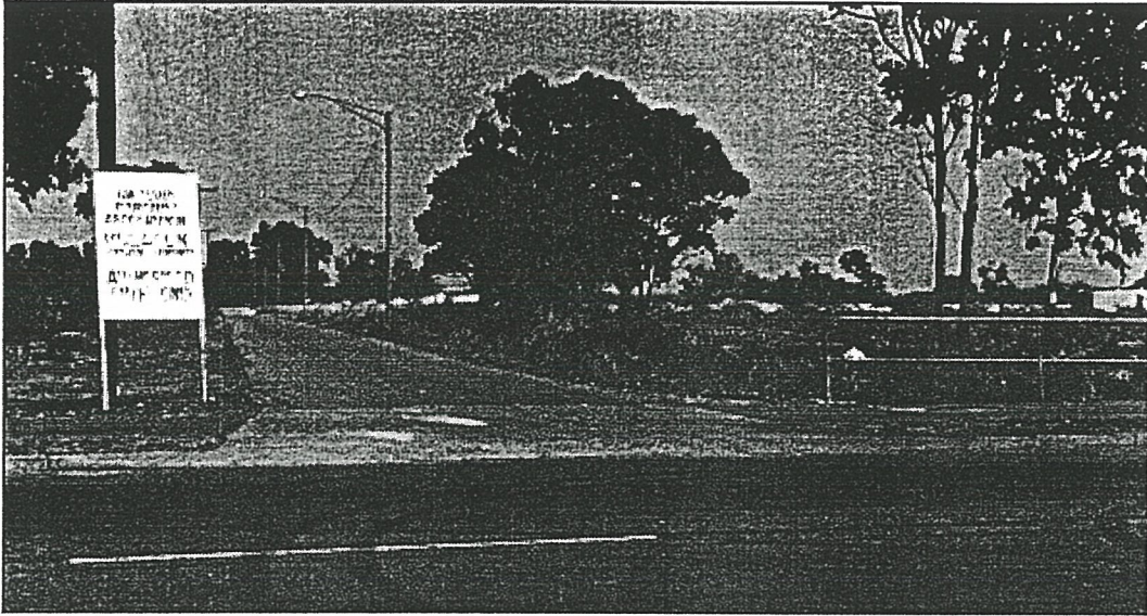
Photograph Twenty-three: The Kulaluk community access road off Dick Ward Drive with an open drain lying along side of it and the Sunset Cove development to its right
